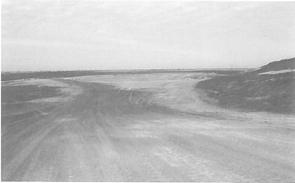
Photo 1: Entrance road to Phase 3A
