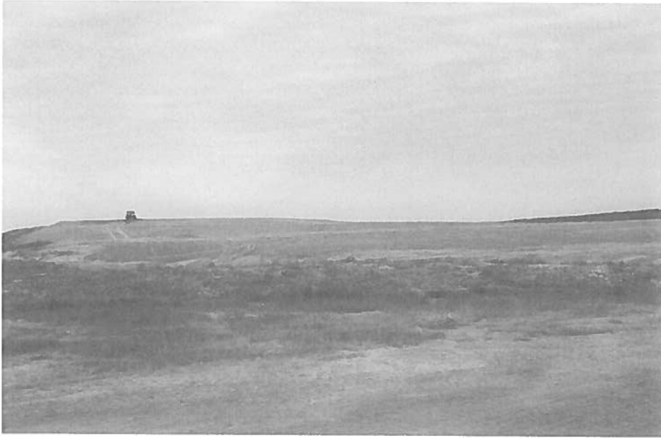
Photo 3: East side of Phase 3A looking west
