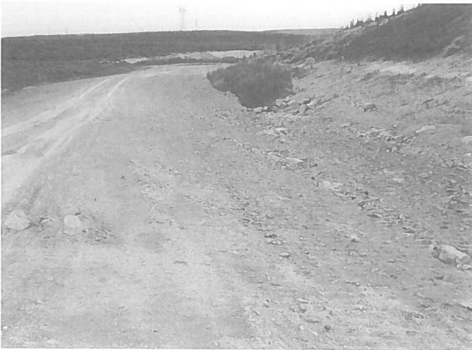
Photo 4: East side of Phase 3A looking east
