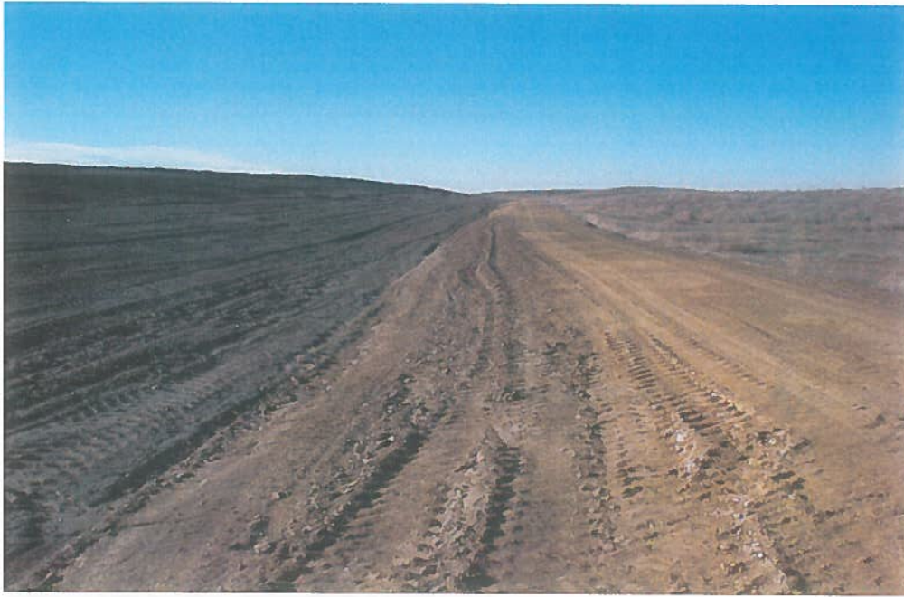
Photo 7: Access road around Phase 3A
