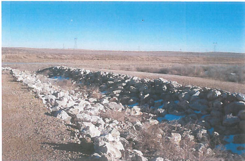
Photo 6: East end of contact water ditch to evaporation basin
